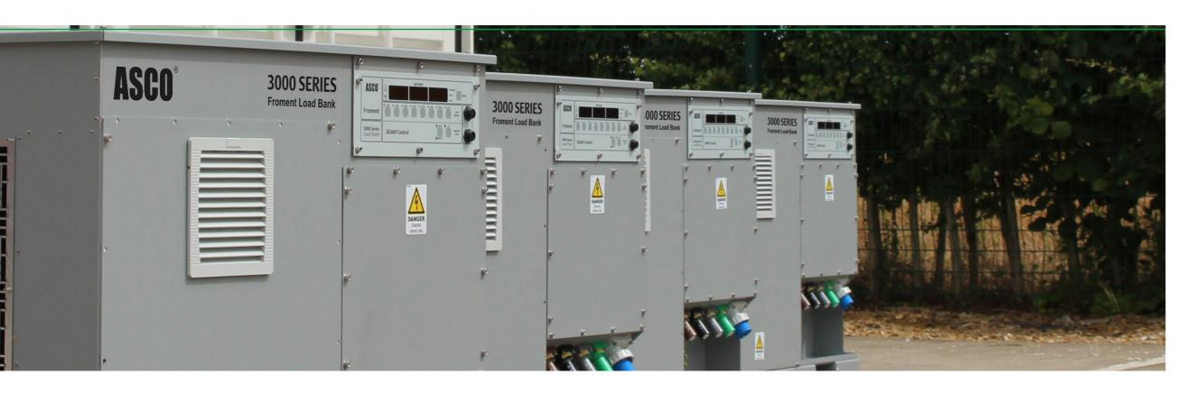
Digital toggle switches are fitted to all SIGMA<sup>LT</sup> load banks and offer simple local control. This method of control is a perfect for quick load tests and useful as a local backup to the SIGMA<sup>LT</sup> hand-held.
